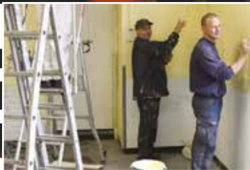
Les services techniques : un service aux actions multiples
